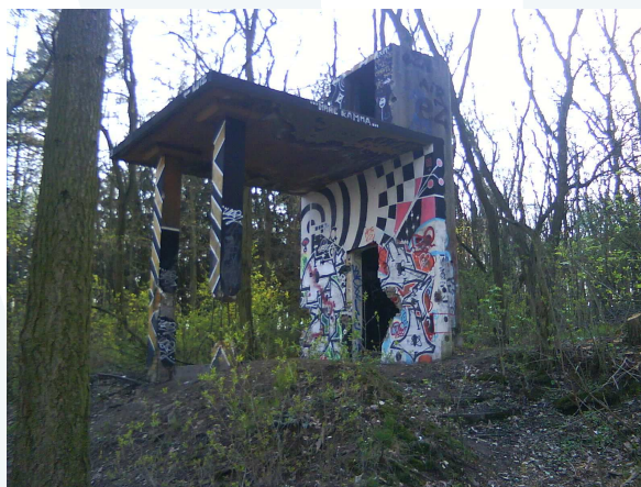
Photo of devastated outlook tower (2010)
